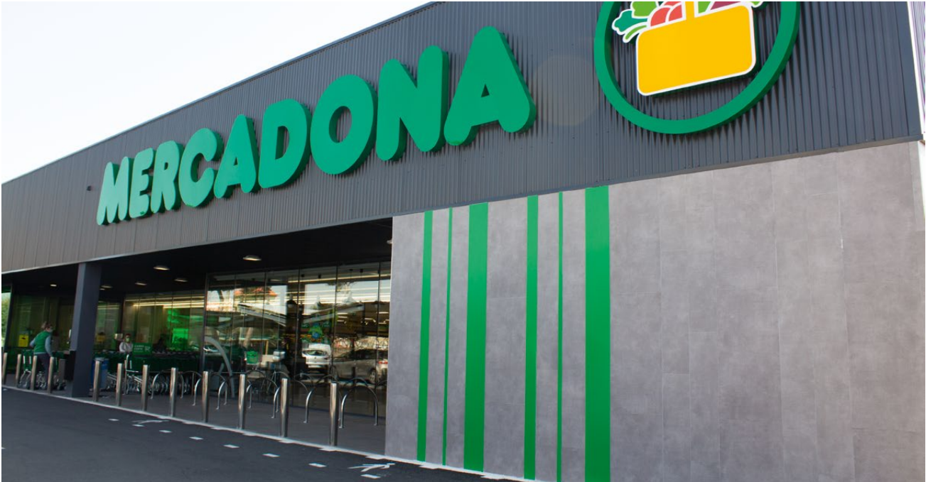
Supermarket Mercadona. Castellón (Spain)
